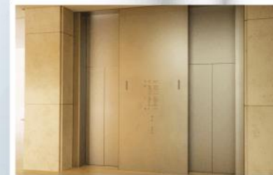
Wall materials around the elevator
